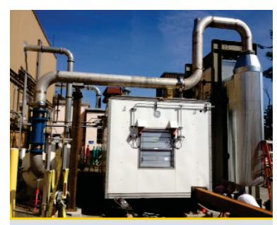
The direct evaporator and supporting equipment installed at the GE test facility. *Photo courtesy of Idaho National Laboratory.*
