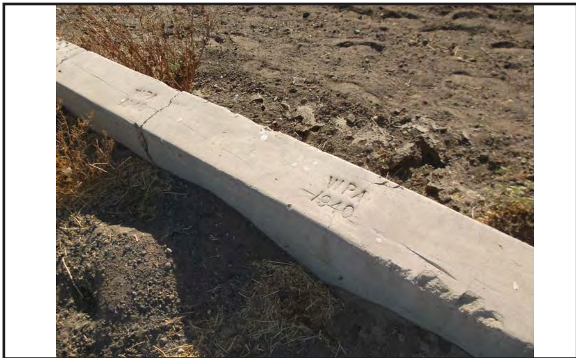
WPA-Era Drainage Headwalls on Dairy Road
