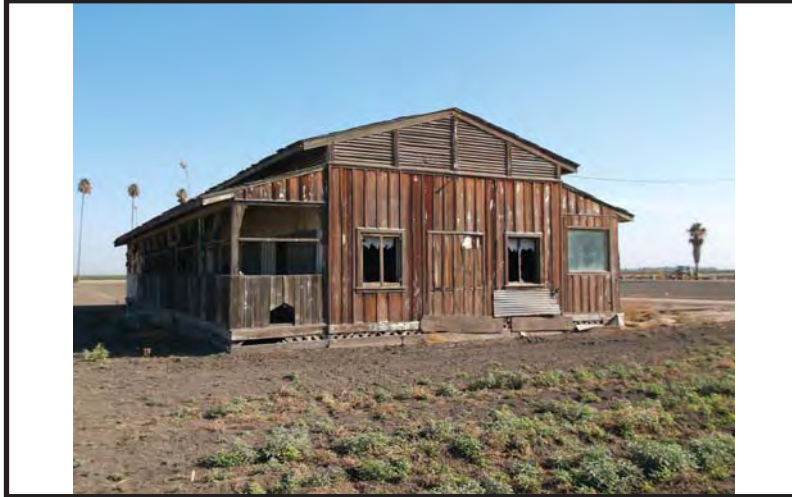
Adohr Farms/Palm Farms Main Residential Building (Building A)
