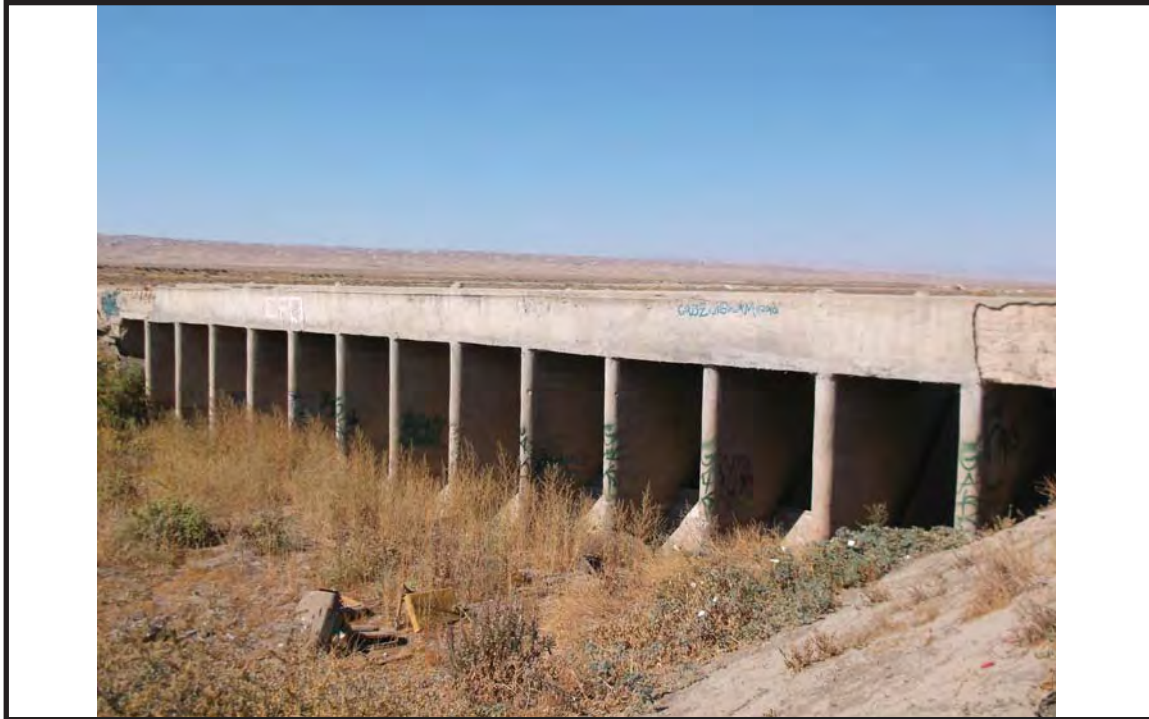
Old Headquarters Weir
