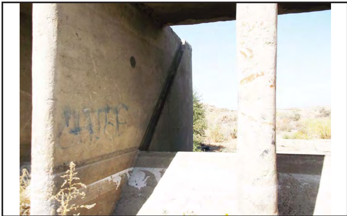
Old Headquarters Weir- View of Channel for Flashboards
