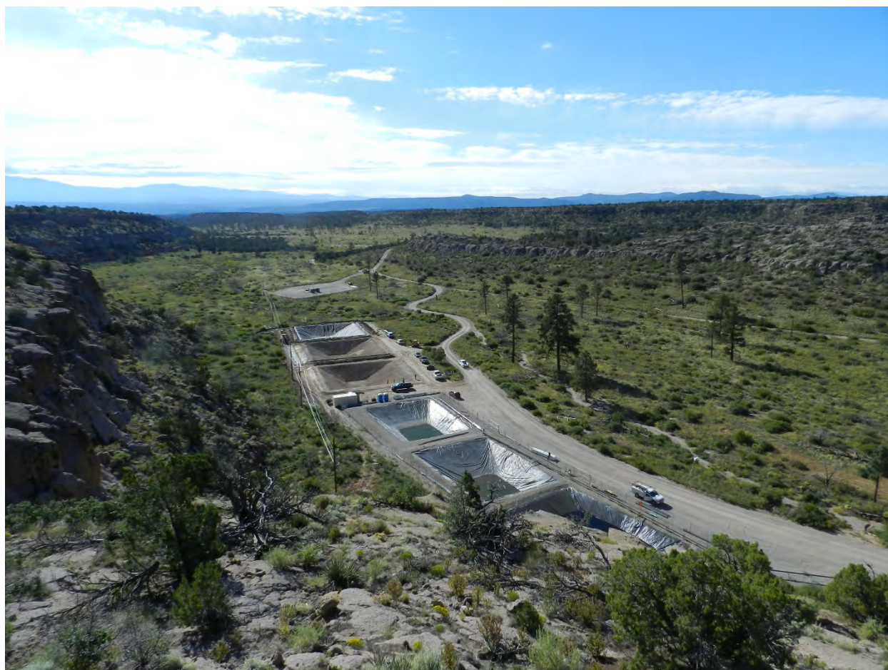
Figure 3-6. Mortandad Canyon featuring storage basins near Well R-28 (facing east from north side of Mortandad Canyon)
