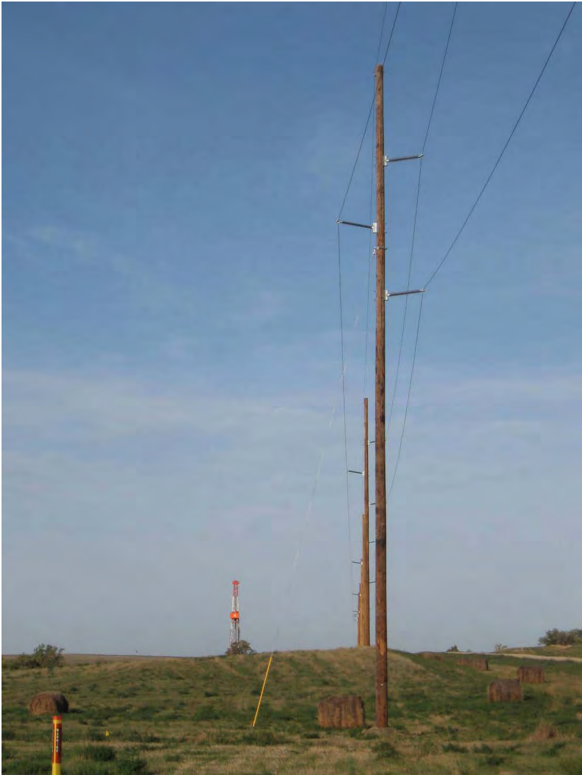
FIGURE 2.2-1: STANDARD SINGLE POLE 115-KV STRUCTURE
