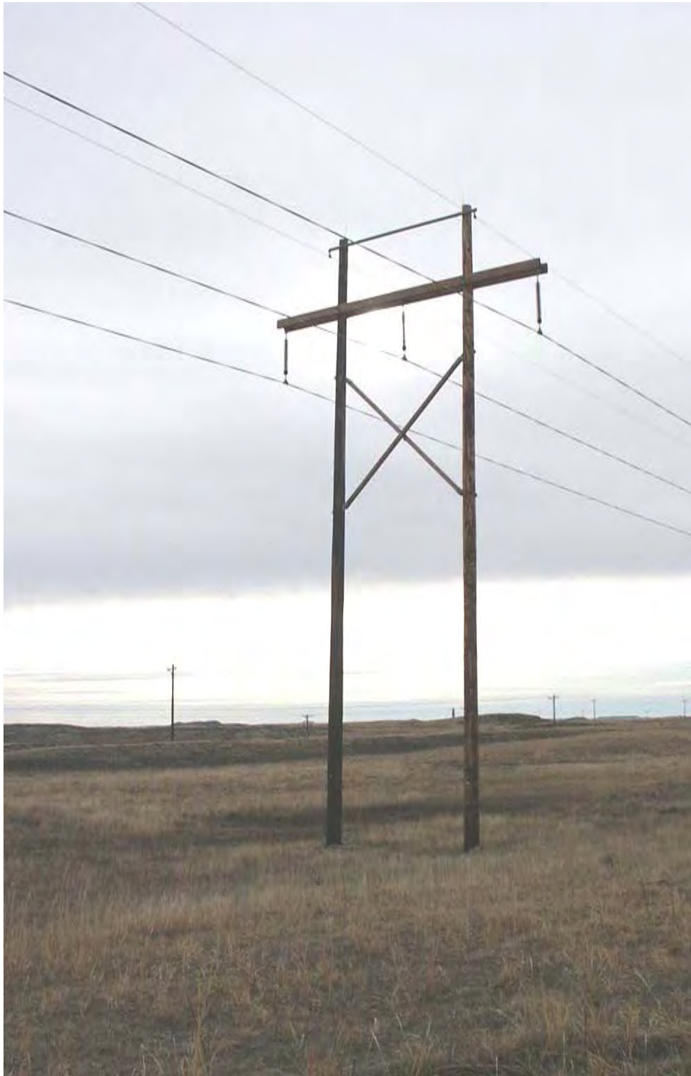
FIGURE 2.2-2: STANDARD H-FRAME 115-KV STRUCTURE
