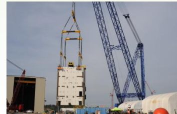
VC Summer Unit 2 CA20 module being removed from module assembly building and set in place (Courtesy of SCANA)
