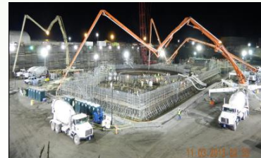
VC Summer Unit 2 cooling tower and Unit 3 basemat placement (Courtesy of SCANA)
