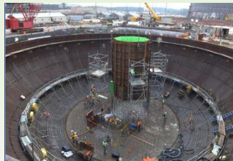
Vogtle Unit 3 CA04 module placement and Unit 3 cooling tower (Courtesy of Georgia Power/Southern Company)
