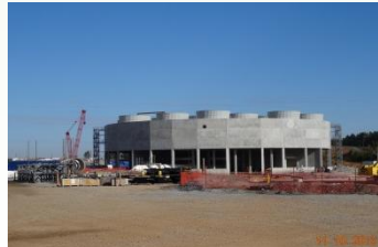
VC Summer Unit 2 cooling tower and Unit 3 basemat placement (Courtesy of SCANA)
