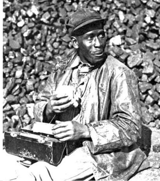
Worker on lunch break War workers were drawn from across the nation. Engineers and scientists, clerks and stenographers, technical personnel and general laborers poured into Oak Ridge to work on the project.
