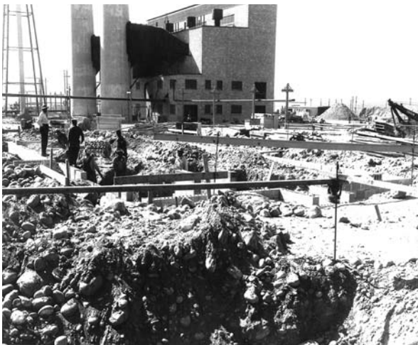
184-B Power House under construction
