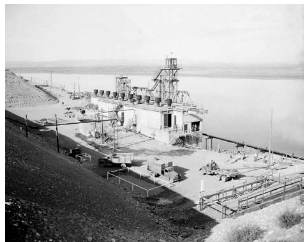
Columbia River Water Pumping Station
