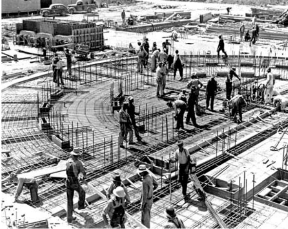
Y-12 Alpha Racetrack under construction
