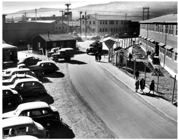
Technical Area 1 Guards stationed at the Main Gate checked cars and passengers for proper identification. Technical area personnel went through another set of gates to enter the laboratory.
