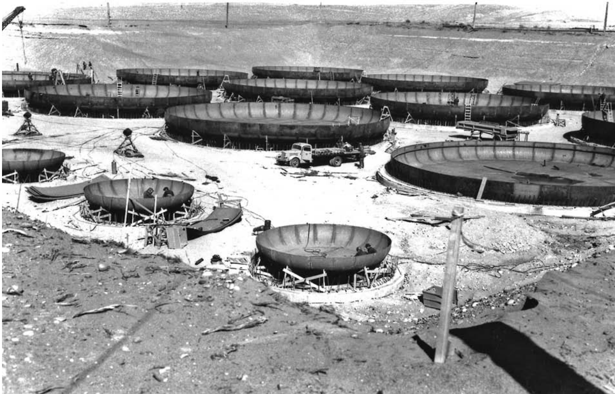
241-T tank farm under construction, early 1944
