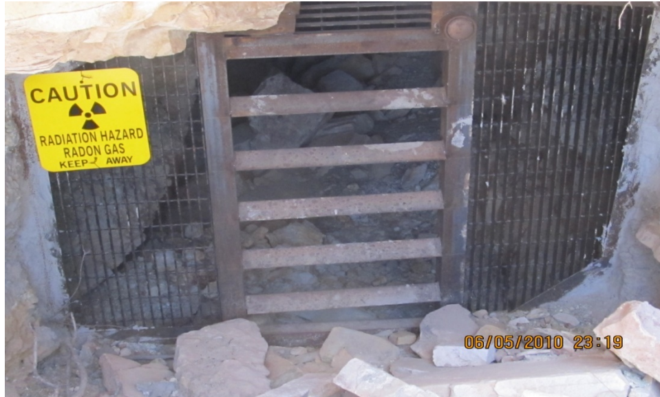
Figure 4. A Mine Adit Closed with a Bat Gate
