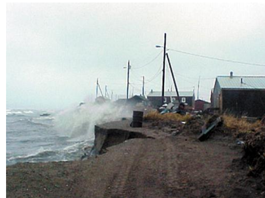
Figure 2-5. Distribution lines in the village of Shishmaref are at risk of damage due to shoreline erosion during coastal storms.
