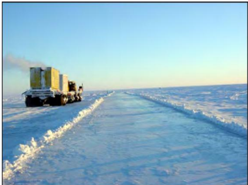
Figure 2-11. A Rolligon (a type of low ground pressure vehicles) prepares the surface of an ice road in the North Slope.
