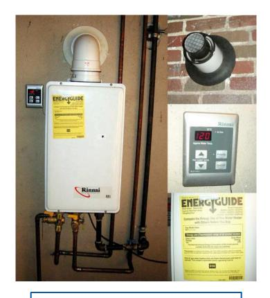
Gas-Fired, Directly Vented, Instantaneous Water Heater
