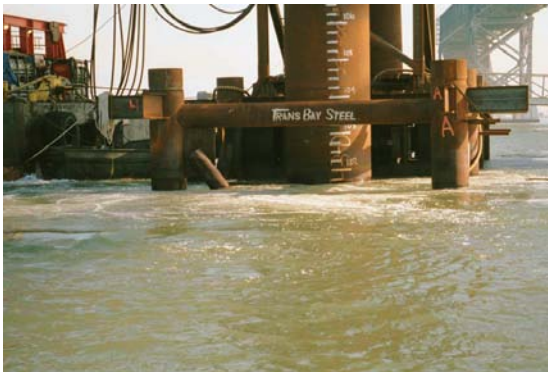
Figure 3-9. Air bubble curtain in operation. Source: Caltrans (2001)
