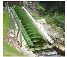
Source: The New England Hydropower Company Figure 1-8. Archimedes screw for hydropower generation
