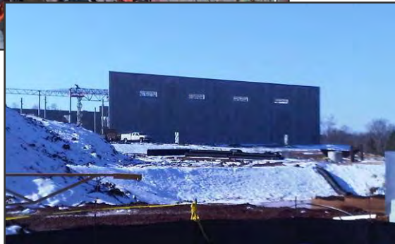
Exterior wall panels are erected
