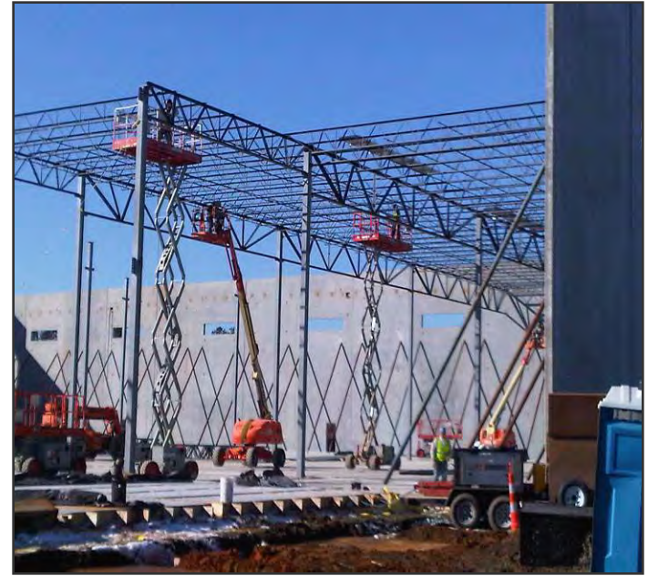
Crews begin installation of the roof steel and structural supports
