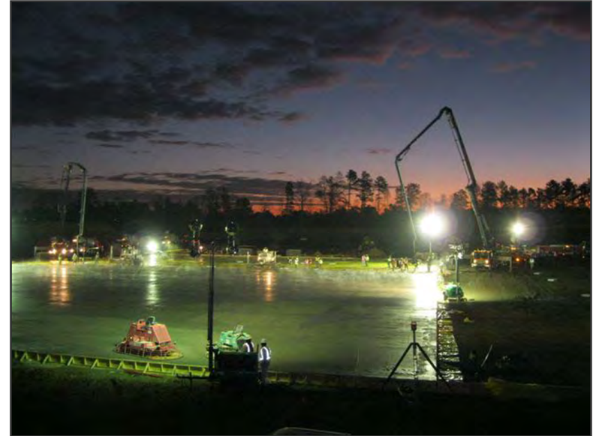
Pouring the concrete slab
