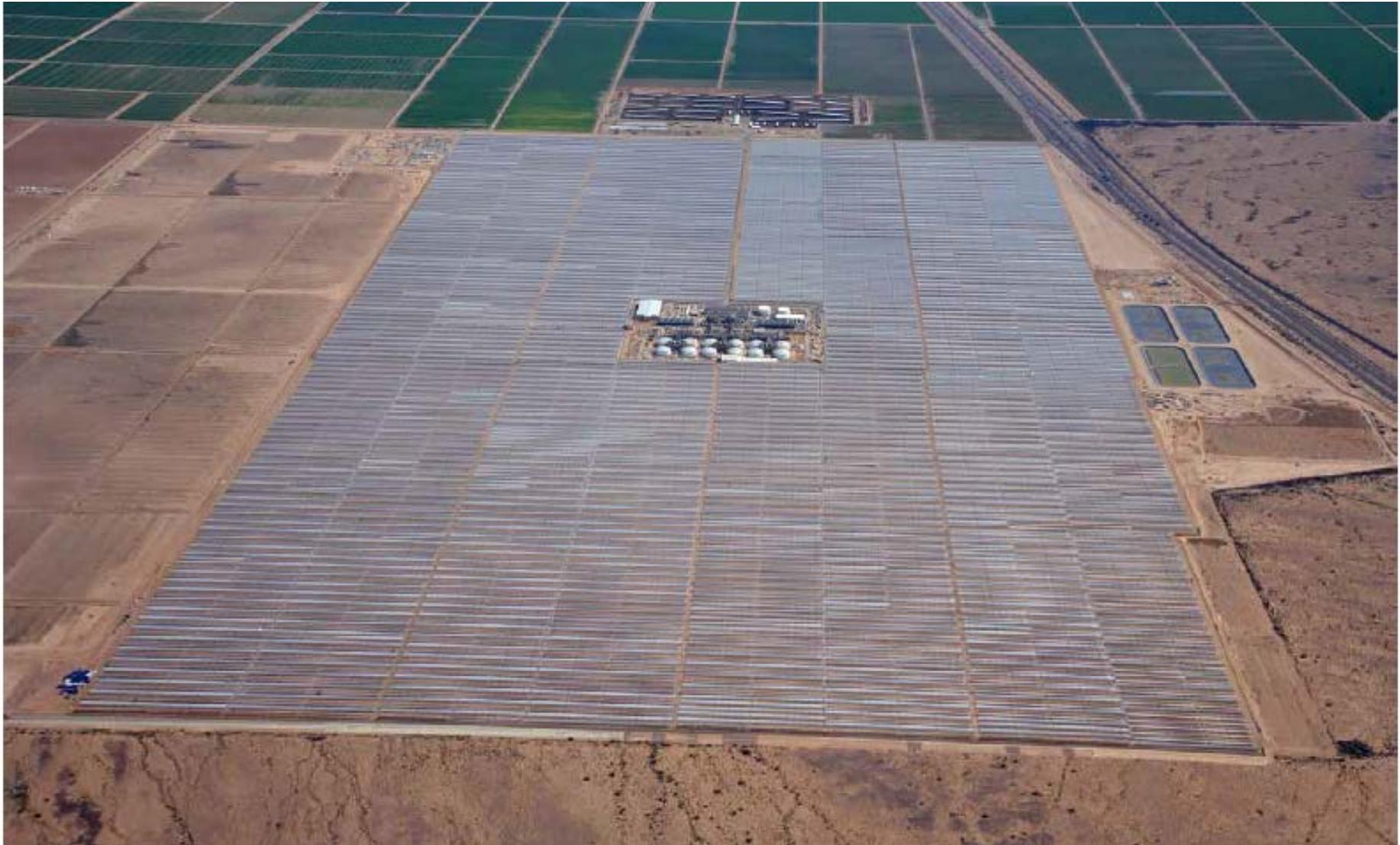
Power Block and TES is located at the center of the solar field
