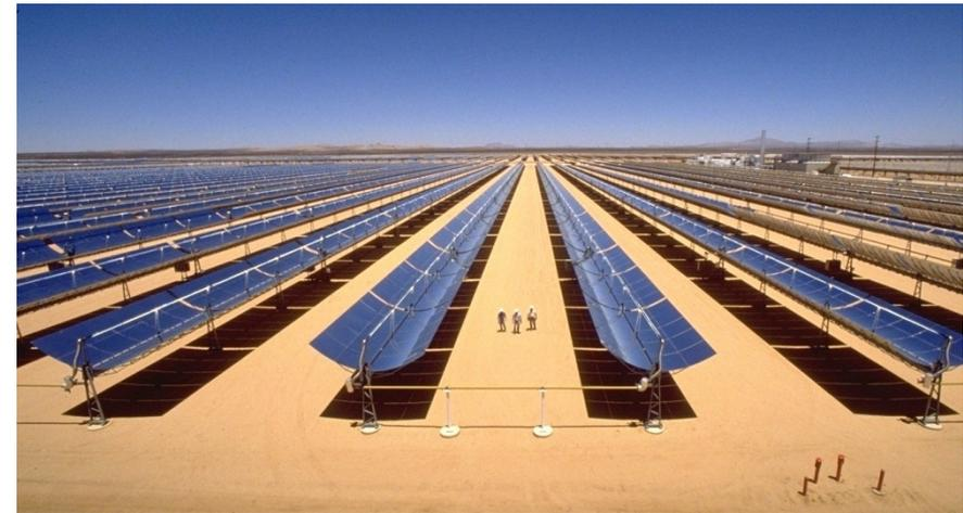
LS-2 Parabolic Trough Collectors, Kramer Junction, CA
