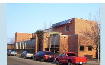
The Larry D. Nelson Engineering Service Building received the first (and smallest) city-owned PV system, at 4.2 kW in size. *Photo from The City of Madison, NREL/PIX* 18356
