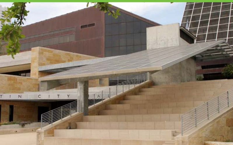
Austin City Hall is a Leadership in Energy and Environmental Design (LEED) Silver building with a 9-kW PV system. Photo from Austin Energy, NREL/PIX 18401
