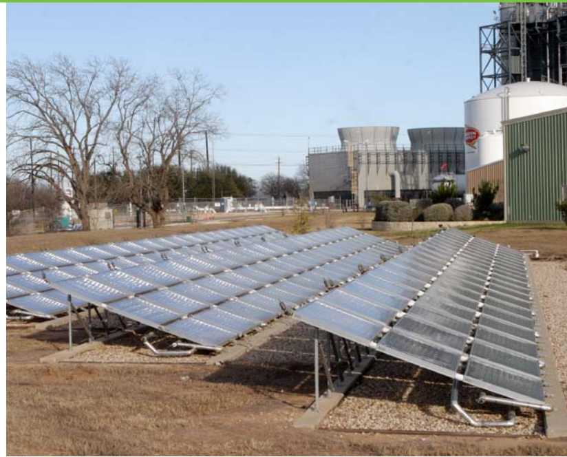
The solar thermal collectors at Austin Energy's Sand Hill Energy Center are used to power an absorption chiller in summer and a heating system in winter. Photo from Austin Energy, NREL/PIX 18402
