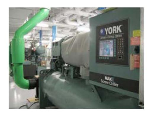
Two (2) 175 Ton (350 Tons total) Chiller Geothermal Heat Pumps for recently commissioned LEED Platinum Building
