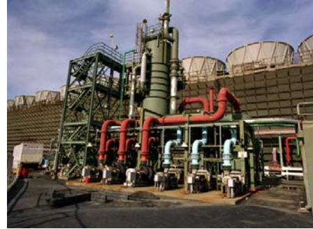
Condensers and cooling towers, The Geysers, being fitted with direct contact condensers developed at NREL
