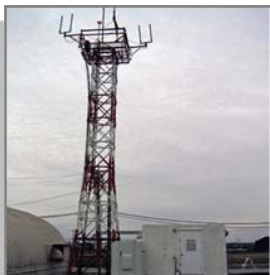
A 1-kW fuel cell system has been providing power for this FAA radio tower near Chicago for more than three years. (Photo courtesy of ReliOn)
