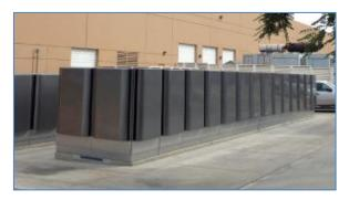
In 2012, Life Technologies installed a 1-MW Bloom Energy fuel cell system at its Carlsbad, California, campus. The fuel cells were installed in an uninterruptible power configuration to protect Life Technologies' labs, freezers, and critical experiments and provide 60 percent of the electricity needs for the facility while reducing carbon emissions by 30 percent. The company previously installed a 1-MW fuel cell system at its Pleasanton, California facility.
