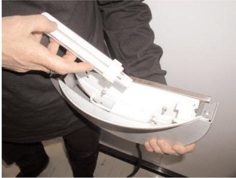
This approach involves the complete removal of the old fixture and replacement with a fixture designed to operate pin-based CFL lamps. The ballast and a socket designed specifically for a CFL lamp are integrated into the fixture. When the lamp expires, only it is replaced. A new fixture system needs to be selected that matches the performance (light output and distribution) of the old incandescent. An electrician most likely will be required for installation and wiring of the new fixture.
