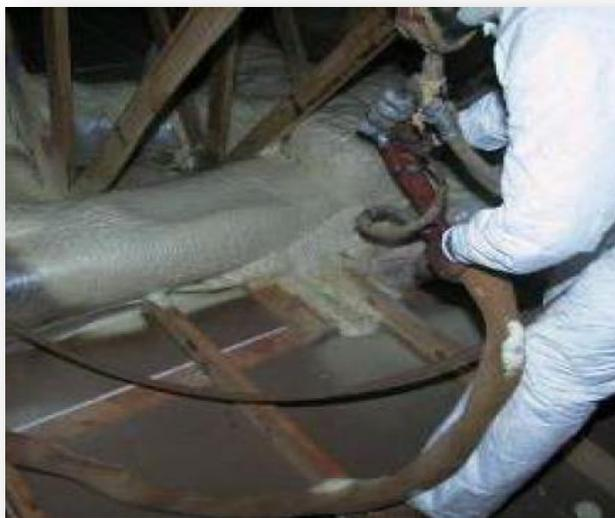
Technique allows ducts installed in a vented attic to meet the code requirements for ducts in conditioned space.
