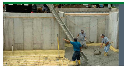
After the basement walls were set but before pouring the concrete basement slab, 2 inches of closed-cell spray foam was sprayed directly onto the 8-inch bed of trap rock, then radiant heat floor piping was laid. The basement walls were then framed with 2x4 16-in. on-center studs set 3 inches in from the concrete walls and spray foam was applied to the concrete basement walls to provide a continuous, air, moisture, and thermal barrier between the foundation wall and the framing.
