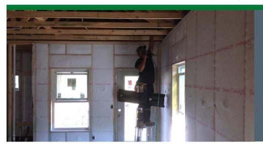
Palo Duro Homes achieves HERS ratings of 48 to 58 by stuffing walls with R-22 of blown fiberglass and carefully air sealing at top and bottom plates, around windows and doors, and at any outlets, wiring or plumbing holes.
