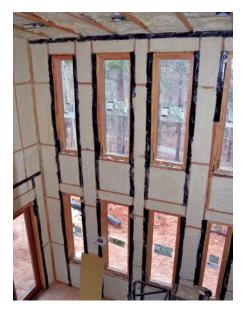
The 2x6 walls were advanced framed to reduce lumber use leaving more space for the open-cell spray foam which provides R-20 worth of insulation in the wall cavities and R-31 on the underside of the flat roofs.
