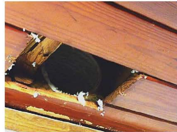
Never Connected Duct
