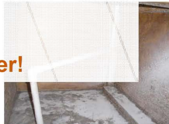
Undersized Return Plenum Open to Walls
