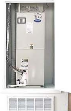
Finished Closet with ≥4" clearance
