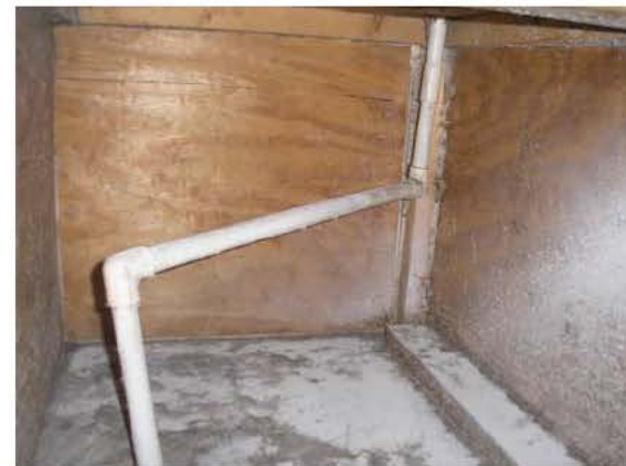
Unsealed, undersized platform return plenum
