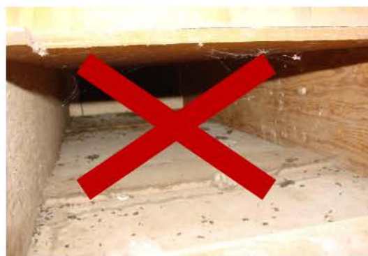
No Building Cavities as Ducts
