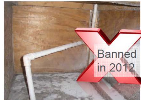
Unsealed, undersized platform return plenum
