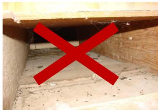
No Building Cavities as Ducts
