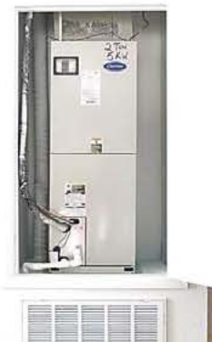
Finished Closet with \geq 4" clearance
