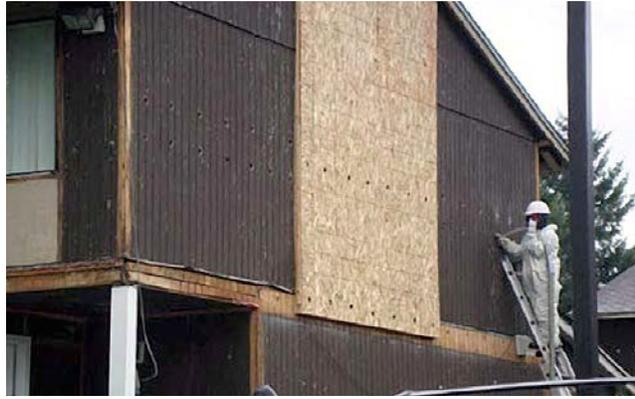
Installation of dense-pack cellulose wall insulation by Arrow Insulation helped reduce heating energy use by more than 40% at the retrofitted Cascade Apartments in Kent, Washington.
