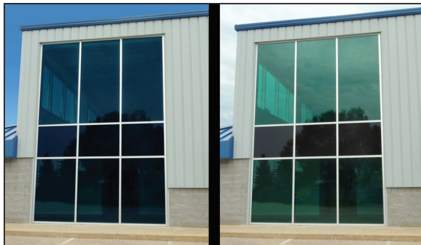
Pleotint's Suntuitive Thermochromic Interlayer Combined with PPG's Azuria® Tinted Glass in the Dark and Light States
