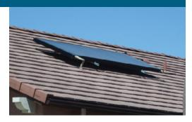
Solar water heaters generate 2,200 kWh/year, enough to recoup the cost of the system within 4 to 6 years.
