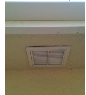
Soffit mounted, filter-back outside air intake.
