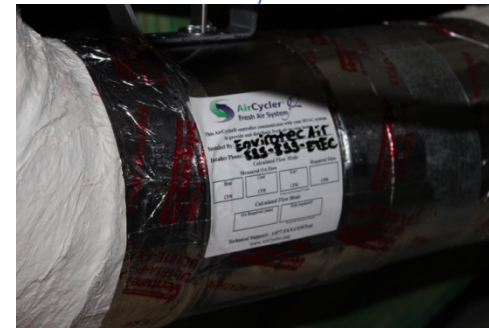
Outside air duct from OA intake to return plenum with electronic damper (connected to the g2K) and manual override damper
