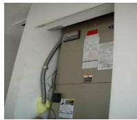
**Left:** This SEER 10 window unit was replaced with a SEER 14.5 central air conditioner, which will save an estimated \$109 each year. **Right:** The new air handler required additional effort to fit into the existing air handler closet space.
