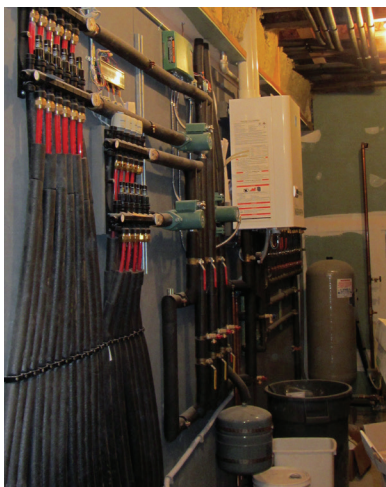
A high-efficiency propane boiler provides hot water for the hydro coil central air heating system, radiant floor heat in the basement, and domestic hot water.
