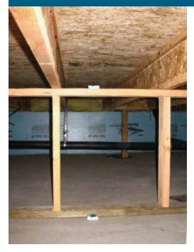
Unvented, insulated crawlspaces are recommended in the cold climate in the eastern and midwestern United States, where high humidity levels can cause moisture problems in vented crawlspaces.
