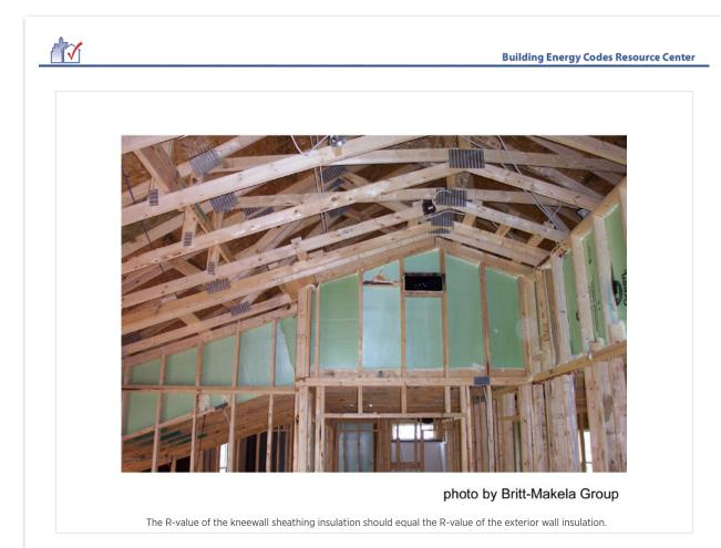
Foam plastic insulation can be installed on the attic side of the attic kneewall (see Figure) to both act as a draft stop between the conditioned house and the unconditioned attic and to increase the insulation R-value of the attic kneewall. Installing such an insulating backing in the kneewall supports the fiberglass batt insulation between framing members, replaces an air barrier, and adds insulating value to the attic kneewall.
