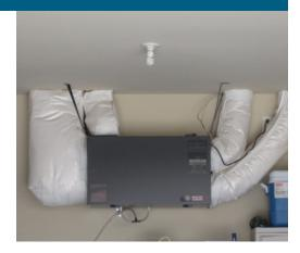
*(top)* Every home is equipped with an energy-recovery ventilator to provide conditioned fresh air throughout the home.
