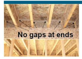
Gaps between garage and conditioned space are properly sealed by carefully cutting and then caulking wood sections to fit between trusses. (*Photo Source: EPA* 2008 "Thermal Bypass Checklist")
