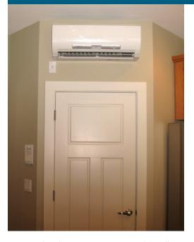
Ductless heat pumps mount to the wall to provide zonal heating and cooling with exceptional energy performance.
