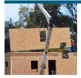
Builder David Sullivan and the South Chicago Workforce worked with Building America on the first structural insulated panel (SIP) home project ever permitted in the City of Chicago. SIPS provide excellent air sealing and insulating properties with fewer seams to caulk and much less thermal bridging than typical stud construction.
