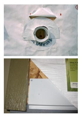
*(top)* This pipe is flashed with flexible flashing. Housewrap is layered shingle style over the top edge of the flashing.
