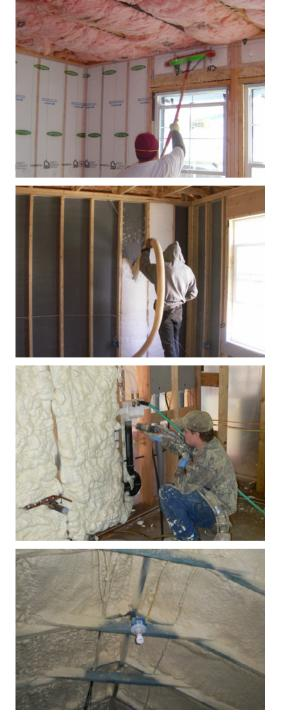
(1) Batt insulation in ceiling. (2) Blown-in insulation. (3) Spray foam. (Photo source: Sam Garst). (4) Spray foam applied along the underside of the roof deck to provide a conditioned and non-vented attic space for ducts and air handlers.
