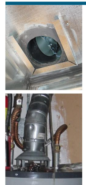
*(top)* This fresh air intake has a mechanical damper to control the intake of fresh outside air into the air handler for distribution via the central HVAC system.
