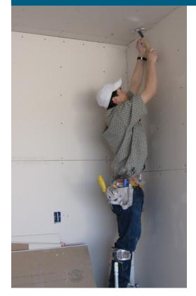
Before the drywalling starts, you should conduct a pre-drywall inspection to test ducts and make sure insulation is properly installed and test moisture levels in framing.
