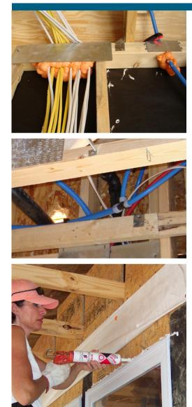
*(top)* Holes in the top plate for wiring are sealed with foam.
