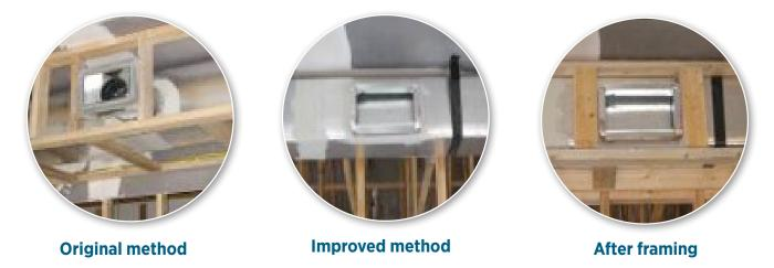
Supply boot comes directly from main trunk, as shown in "improved method" rather than connecting boot to trunk with a length of flex duct, as shown in original method. Thus duct chase can be narrower.
