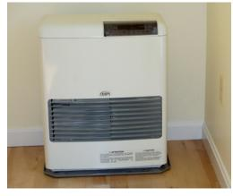
The homes are so well insulated that a 10,200-Btu gas-fired space heater on the main floor, (shown in wood cabinet in top photo and alone in bottom photo), provides all the heat needed.
