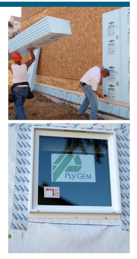
(top) When rigid foam insulation is applied to the exterior side of the wall cavity under the cladding, with seams taped and glued down, it acts as a vapor barrier, preventing moisture in brick and stucco finishes from being driven inward during drying. It also serves as an air barrier and rain screen, and during the heating season, it maintains the temperature of the wall cavity above dew point, to prevent condensation. (Photo Source: S+A Homes)
