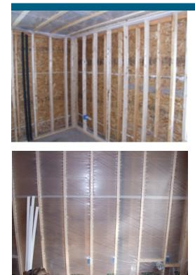
*(top)* The double-stud wall consists of two 2x4 16-inch-on-center framed walls set 5 inches apart.
