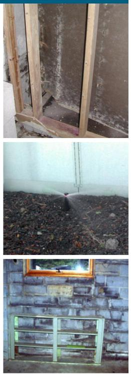
(top) When moisture is trapped inside walls, mold can grow unchecked, causing damage to the walls and health impacts for the occupants. (Photo source: EPA; photo by Terry Brennan)
