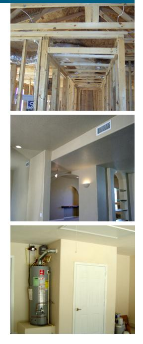
(1) One technique for placing ducts in conditioned space is to run a duct chase in a dropped ceiling down the main hallway of the house with registers off the sides for each room. This technique allows for compact duct design.
