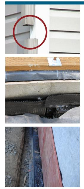
(top) Make sure the downspouts are continuous to the ground and extend to at least 3 feet from the house. Install flashing at the roof valleys and edges and install rain gutters to guide water off the roof and away from the house. (Photo Source: EPA, photo by Terry Brennan)
