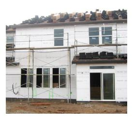
Taped rigid foam insulation can serve as a drainage plane, air barrier, and vapor barrier as well as a thermal boundary behind a stucco cladding. If using housewrap instead, never apply stucco directly to plastic housewrap. Provide a drainage space to prevent wetting of the housewap or use two layers of textured building paper.
