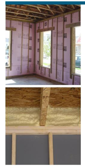
*(top)* Masonry walls are insulated with interior rigid insulation.
