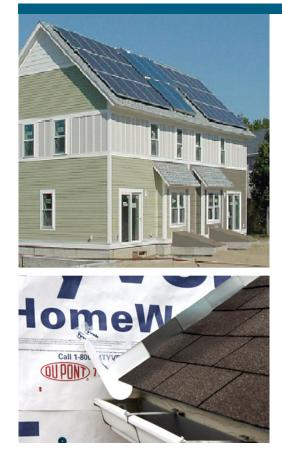
(top ) RDI used a basic roof shape on its homes in Greenfield, Massachusetts, which minimizes the need for complicated flashing and provides the added benefit of more space for photovoltaics and solar water heating panels (*Photo Source: RDI*).
