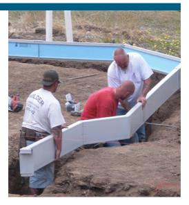
Davis Energy Group of the CARB Building America team developed a method for insulating slab perimeters. The method, which is commercially available, uses termiticide-treated rigid foam insulation encased in PVC as the form for the concrete foundation. In cold climate locations, the forms can be stacked to provide deeper protection against frost (Personal communication with David Springer, Davis Energy Group, 11/10/10).
