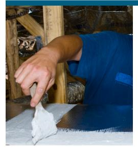
*(Bottom)* Mastic provides the most reliable duct sealing method. Ducts should be located in conditioned space. *(Photo source: BAIHP)*
