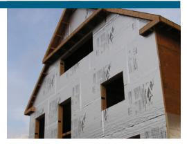
Nelson Construction of Farmington, Connecticut, uses two inches of foil-faced polyisocyanurate insulating sheathing taped at the seams for an insulated air sealed exterior that is finished with Tyvek house wrap and vinyl siding.
