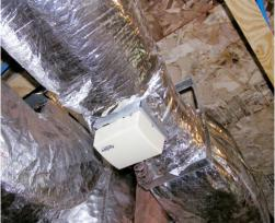
Nelson Construction attached a fresh air intake with a timed mechanical damper controller to regulate fresh air flow into the return plenum of the HVAC air handler. The damper can be set to open allowing fresh air to be pulled into the air handler by the air handler fan, also operated by the timer. This draws fresh air into the house at regular intervals. When combined with timed exhaust fans, this provides low-cost balanced ventilation.
