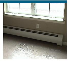
Hydronic heating in condominiums in Aspen, Colorado, uses water that is preheated by solar thermal panels, than heated by a gas boiler, and distributed via baseboard radiators.
