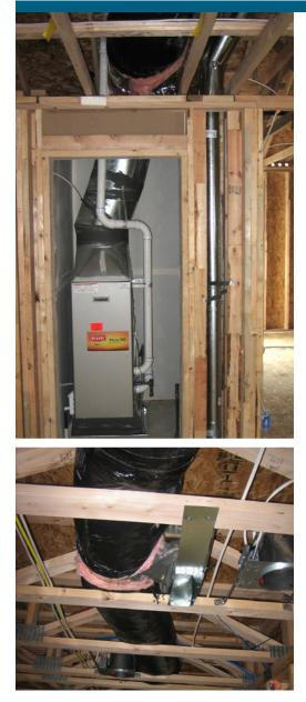
(Top and Bottom) These Building America builders run ducts through open-web floor trusses to keep the ducts in conditioned space (shown here). Open-web trusses allow subcontractors the flexibility to run plumbing, electrical, and ductwork easily between floors, with little to no "trade damage" or "trade fighting." Air handlers are located in conditioned space in the home or in an air-sealed closet in the garage.
