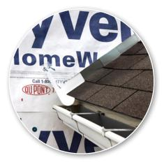
**STEP 6** Install house wrap; cut the house wrap to fit over the self-adhesive flashing and sidewall flashing.
