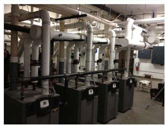
2011 Replacement with (4) high-efficiency 500,000 BTU, separate controls, insulated pipes.
