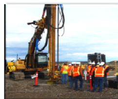
Workers with small business Hayward Baker, Inc., injected cement-based grout into 21 buried waste locations to stop rain and snow melt from infiltrating the contaminated waste produced during historic operations at the Idaho site.
