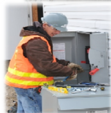
DKM subcontractor installing electrical systems for construction field trailer
